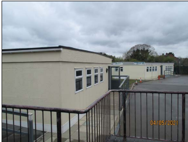
Mobile units to be demolished
