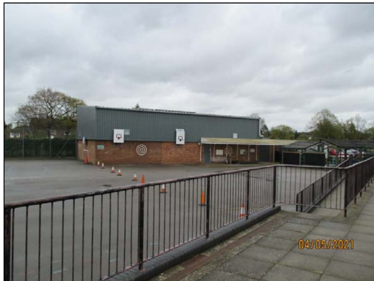
Sports Hall to be demolished
