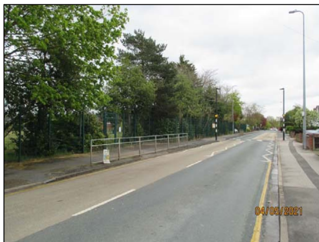
School frontage on Skellingthorpe Road
