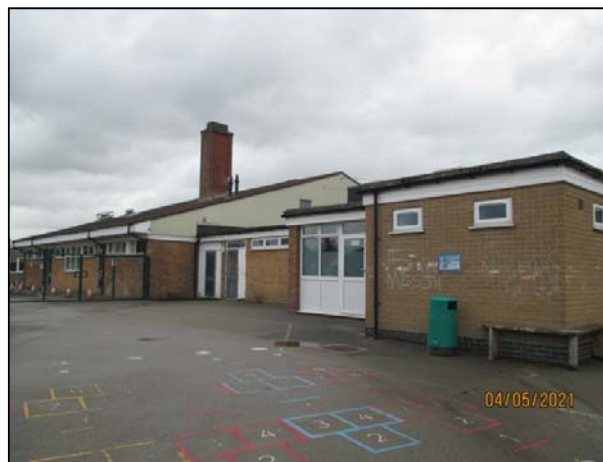
Block 2 & 3 to be demolished
